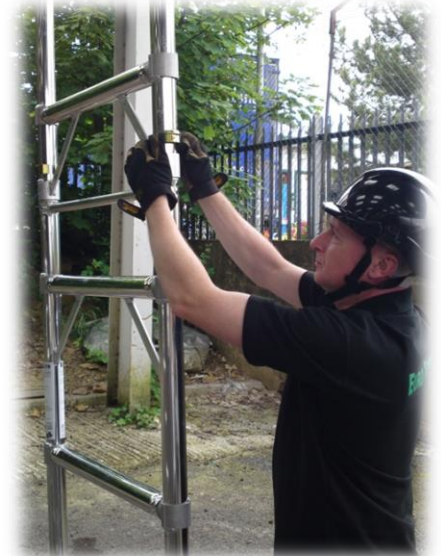
4. Engage Interlock Clips.
