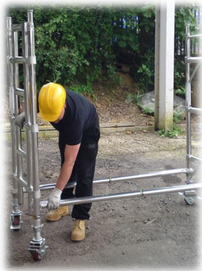
2. Klik in 2 horizontal braces to the vertical member of the frames, as low as possible, below the 1 st rung.
