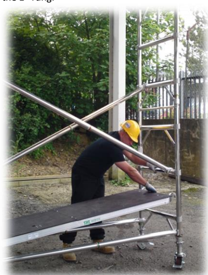
6. Fit temporary platform to the 1 st rung and level base.
