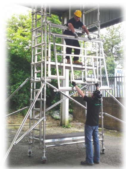
12. Safely pass up the next set of AGR frames as shown.
