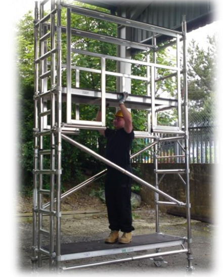
8. Position the trapdoor platform to the appropriate rung (Trapdoor facing the ladder section) 1 rung above the bottom section of the AGR frames.
