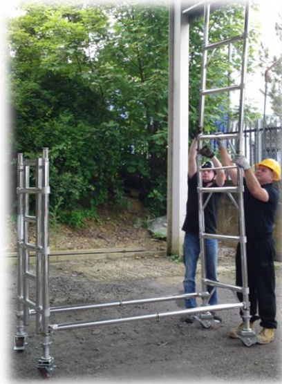
3. Add next level frames – according to your kit list.
