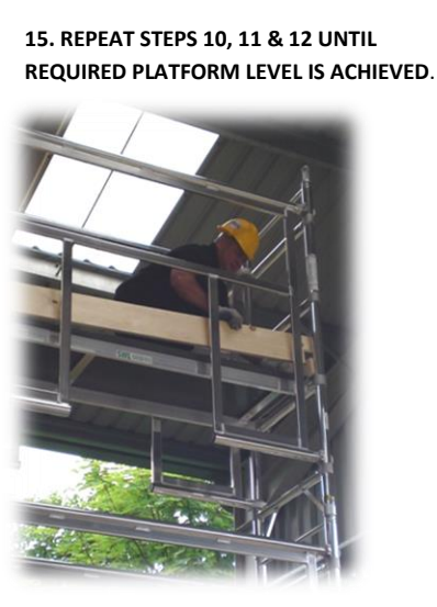
16. Fit toeboards in the correct position.
